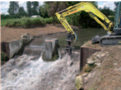
Weir during the works: return to free-flowing conditions - 2008
