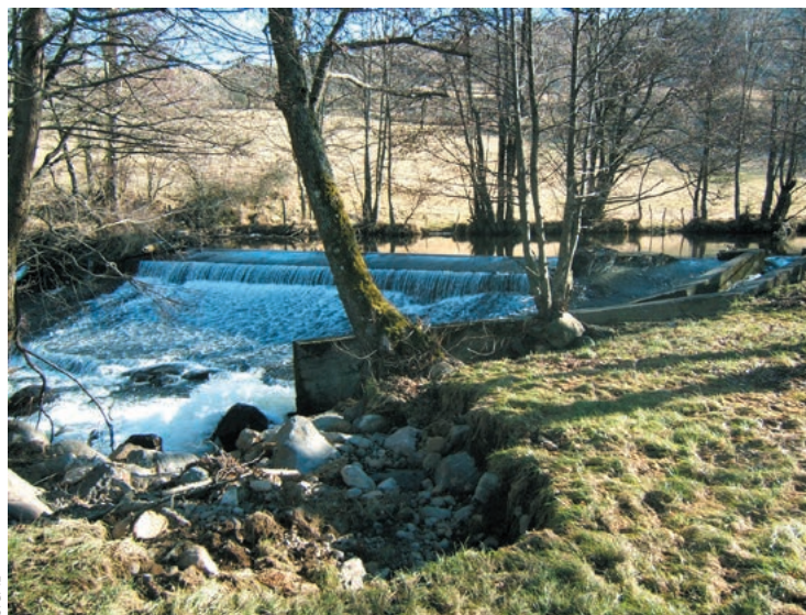
View of the weir before its removal.
