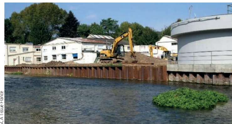
Filling in the factory leat following the removal of the Plis weir (2014).
